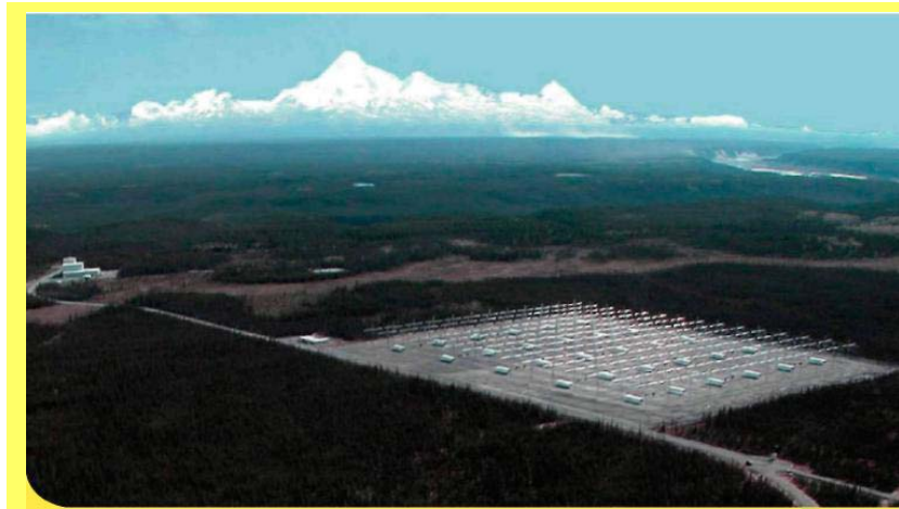
Fig. 25: HAARP location and construction.
