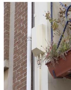
Microcell antennas are a lot smaller than macrocell antennas and can often be disguised as building features.
