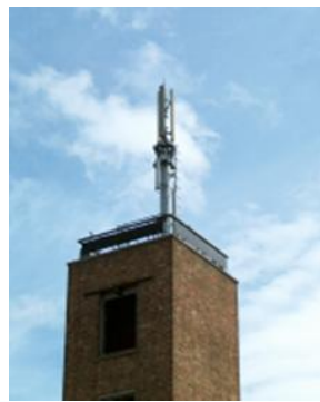
Mast on existing structure
