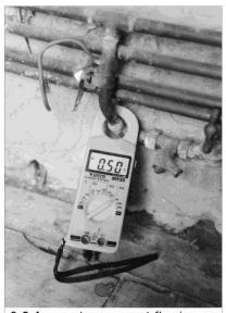
0.5 Amps stray current flowing on incoming main cold water pipe
