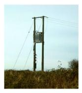
The fields from these transformers fall off very rapidly and are usually negligible further than 3 metres away - the fields from the overhead wires are usually more concerning, and the  $11~\rm kV$  wires should not pass within  $20~\rm metres$  of the house.
